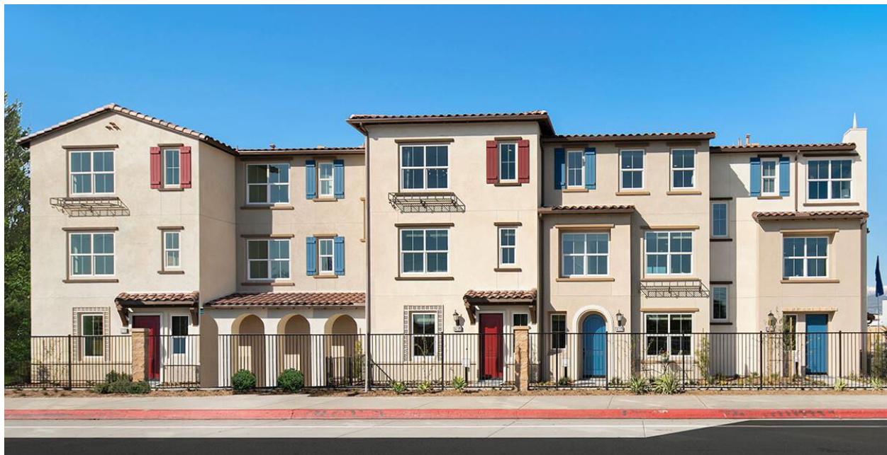
Palmera Mixed Use Project includes 23 townhomes and reuse of the historic Vineland Substation No. 21, a former facility used by the Pacific Electric Railway, 2020.
