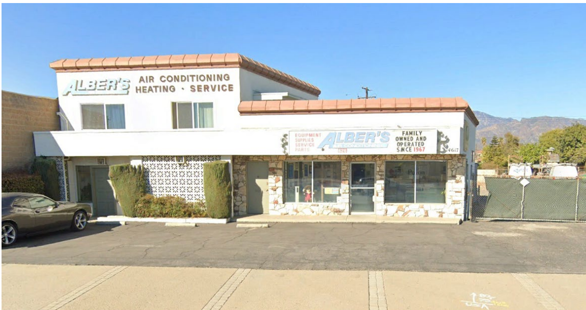
Site of Approved Project – 14617 Ramona Cesar Chavez Foundation Project, Existing Conditions
